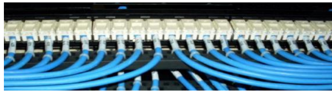
Figure 5.3 - Patch panel (horizontal guide).
