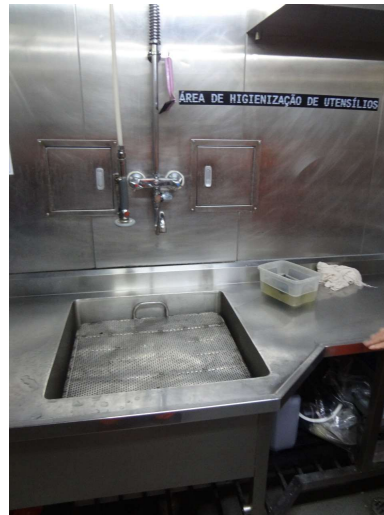
Figure 10. Sink with support.
