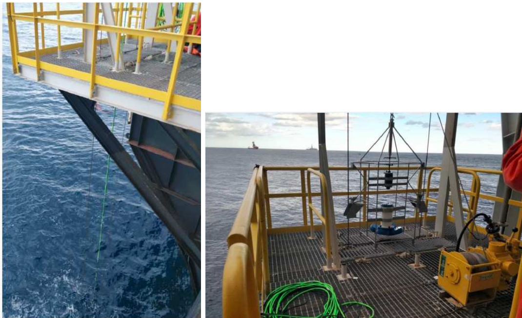
Figure 2: Advanced deck structure as a trapdoor. [Left] Sensors in operation; [Right] Sensors on the deck for maintenance.
