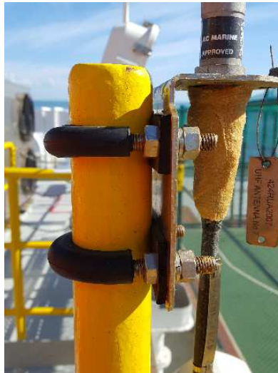
Figure 10: Insulation to avoid galvanic corrosion
