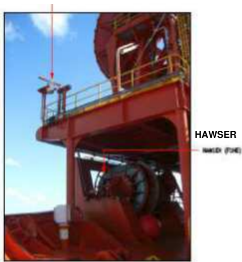
LRMS ANTENNA (FORE)
